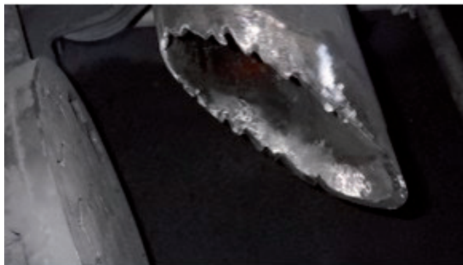
Figure 6 Secondary cyclone dipleg erosion
