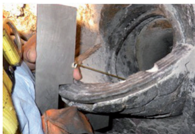
Figure 4 Feed nozzle measurement prior to installation
